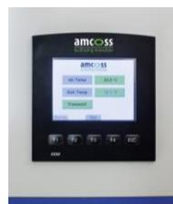
// The controller with a touch screen is located on the top cover of the chiller. It manages the communication to the tool
